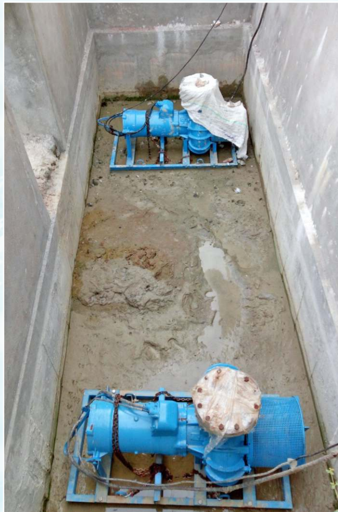
Submerged CF Pumps can be simply bottom rested in to existing suction pits.
